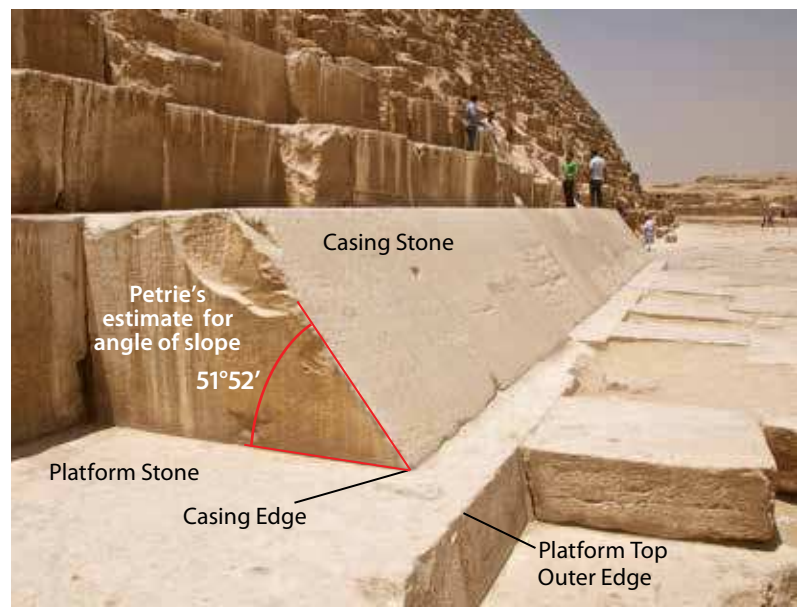
Casing and Platform Stones. Near the corner of the north side the angled casing stones sit upon platform stones. The lower, outer edge of the casing and the top, outer edge of the platform provide the best places to measure the Pyramid's lines. Petrie estimated the angle of the casing slope to be 51^{\circ} 52' \pm 2' minutes. Photo by Mark Lehner.
